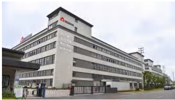
高新区工厂 High-tech Zone Factory
